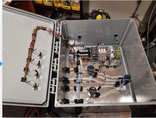
Sample influent Stream switching
